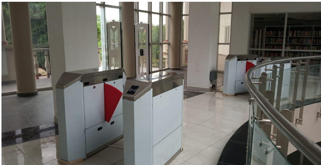
Flap Barriers (For entry and exit to the library)
