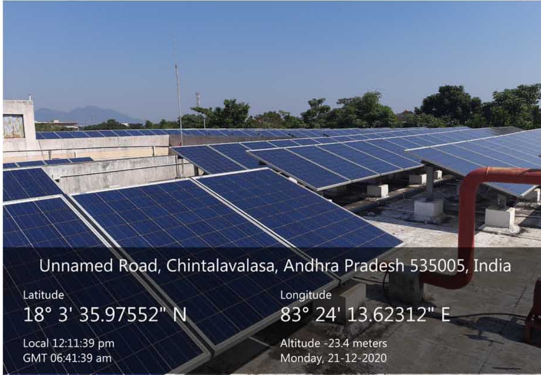
95Kwp Plant located on rooftop of MECH department and associated Inverters
