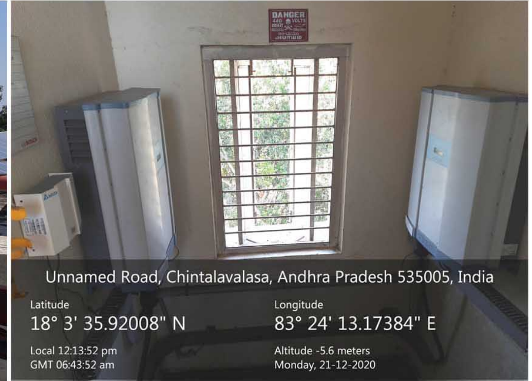
95Kwp Plant located on rooftop of MECH department and associated Inverters
